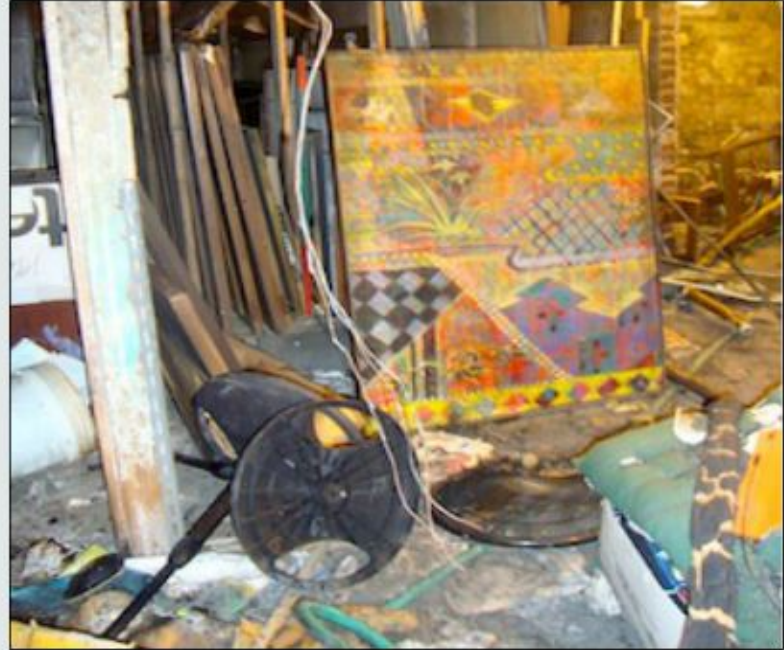
House Fire Philadelphia PA 2014
