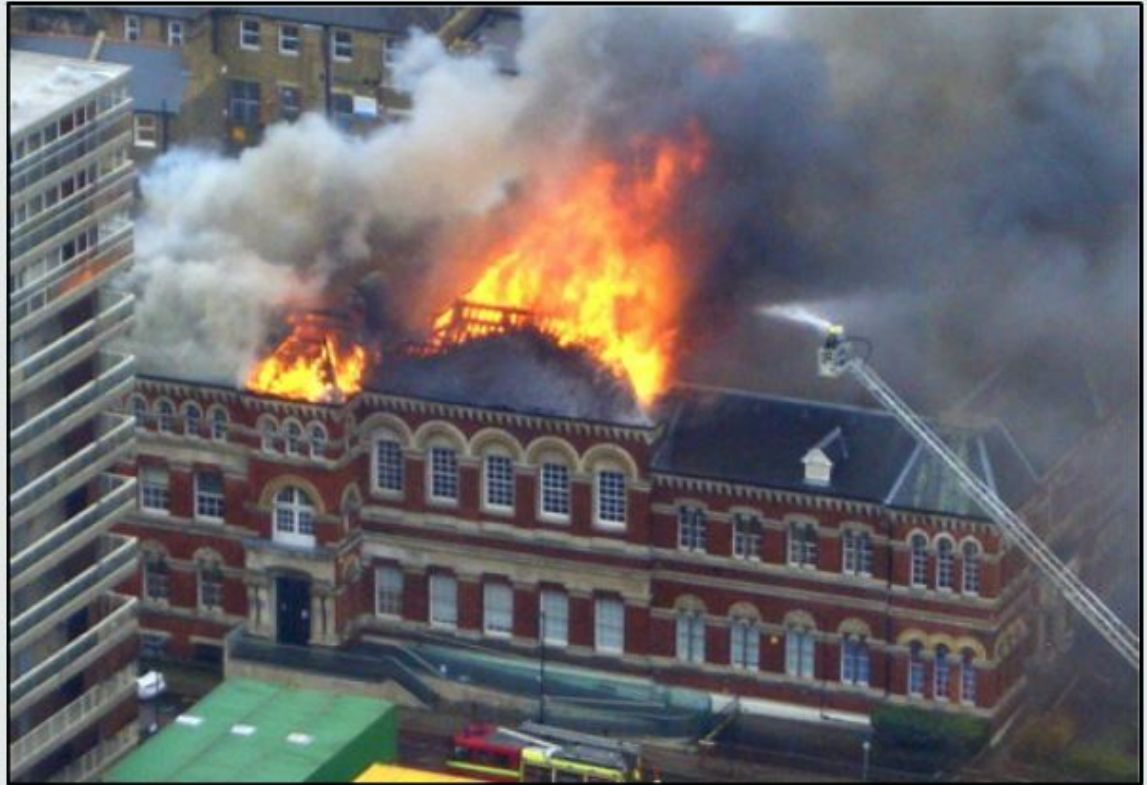
Cuming Museum Roofing Construction Accident London 2013
