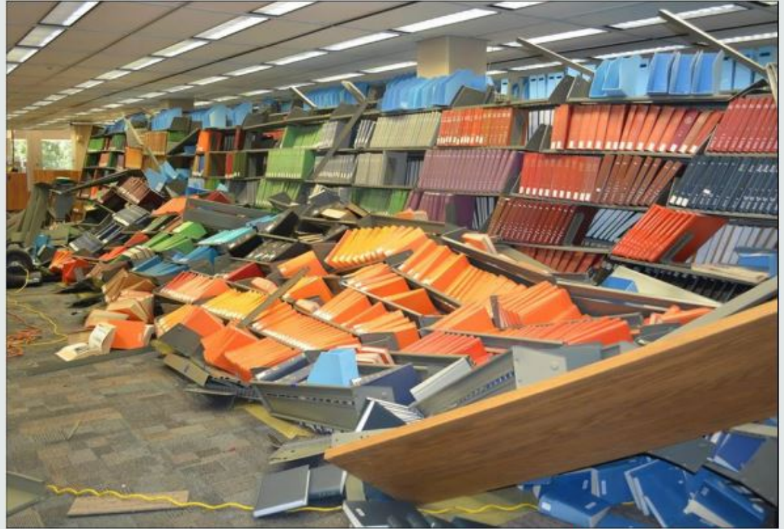
University of Texas Stack Collapse, 2015
